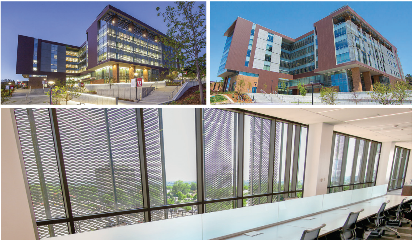
SJ Quinney Law Building designed by the Smith Group - Parallel sunshade using APEX03 mesh, interior and exterior view
